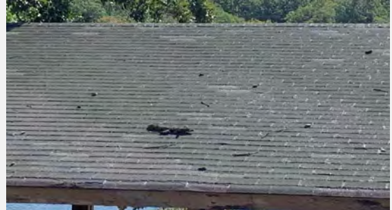
Recommended to, at a minimum, replace roof shingles with ribbed
