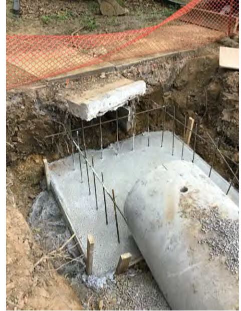
FCO #2 Drainage culvert connection found during construction. Contractor was instructed to correct this issue, as the site was already prepped for the work.
