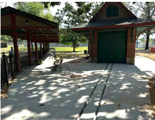
FCO #2 Improved entrance to Creekmore Express to comply with ADA requirements, reconfiguration of the drain system to mitigate pooling of stormwater at the entrance and around the train depot, and installation of electric conduit to eliminate the need to run extension cords on the ground and/or through trees for holiday displays.
