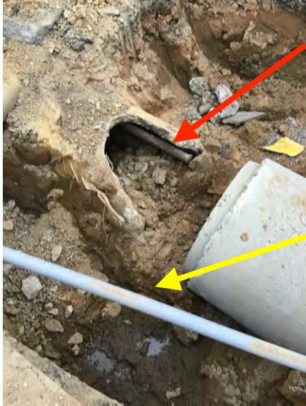
FCO #1 Existing electrical conduit for the miniature golf building within the storm drainage pipe.
