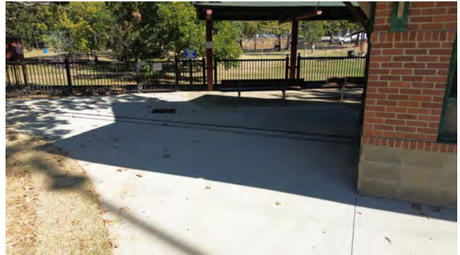
FCO #2 Improved entrance to Creekmore Express to comply with ADA requirements, reconfiguration of the drain system to mitigate pooling of stormwater at the entrance and around the train depot, and installation of electric conduit to eliminate the need to run extension cords on the ground and/or through trees for holiday displays.
