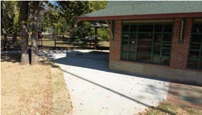
FCO #2 Matching grade to the sidewalk west of the train depot was not ADA compliant. This section was removed and a new, ADA compliant section was poured.
