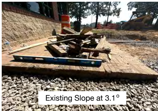
FCO #2 Matching grade to the sidewalk west of the train depot was not ADA compliant. This section was removed and a new, ADA compliant section was poured.
