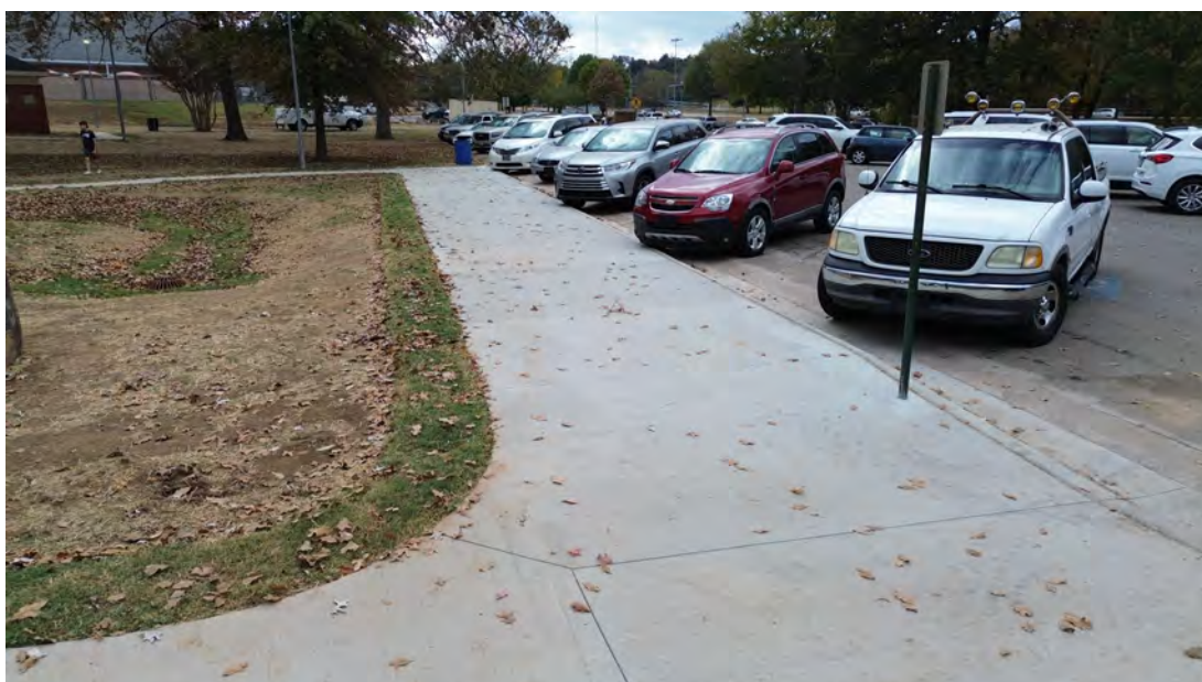
Completed project with curb and gutter in lieu of reinstalling concrete parking blocks.
