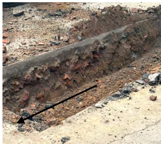
Mix of Whole and Fragmented Brick Subbase
