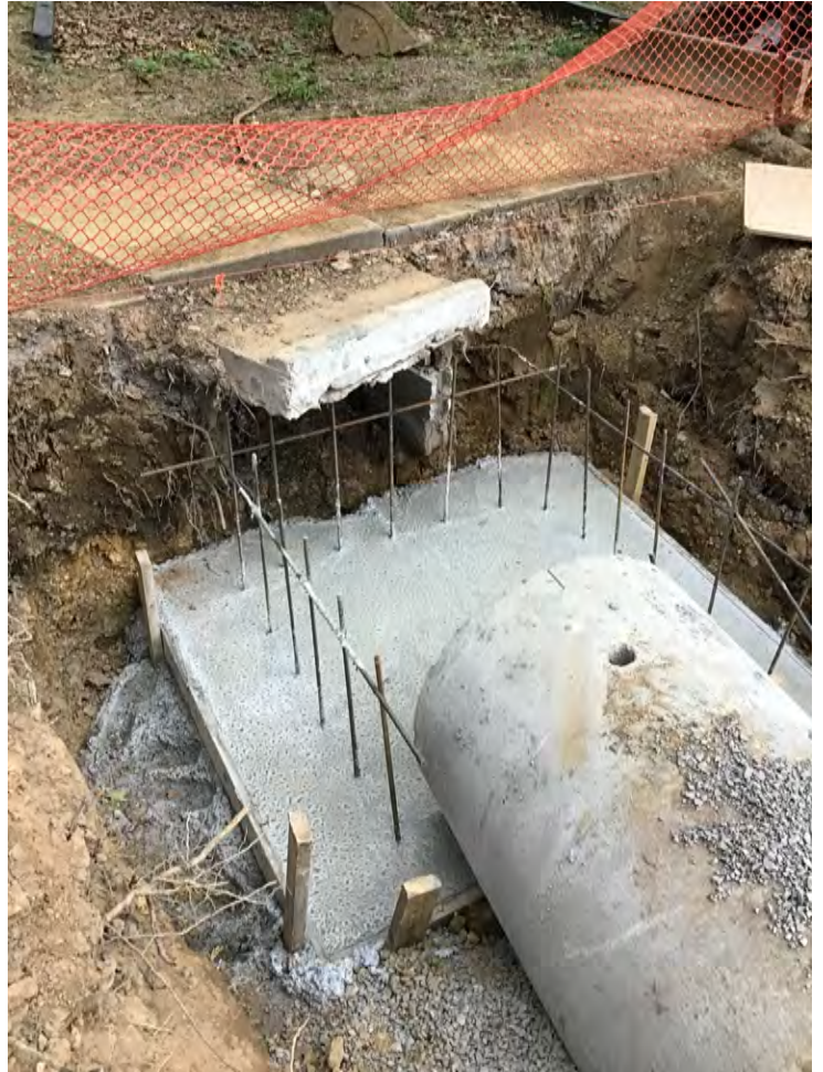
Eastern drainage culvert connection
